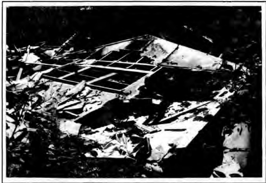
Figure 17. The ruins of the Durand Restaurant/Parker Bar, 1993. The view is looking northwest.
